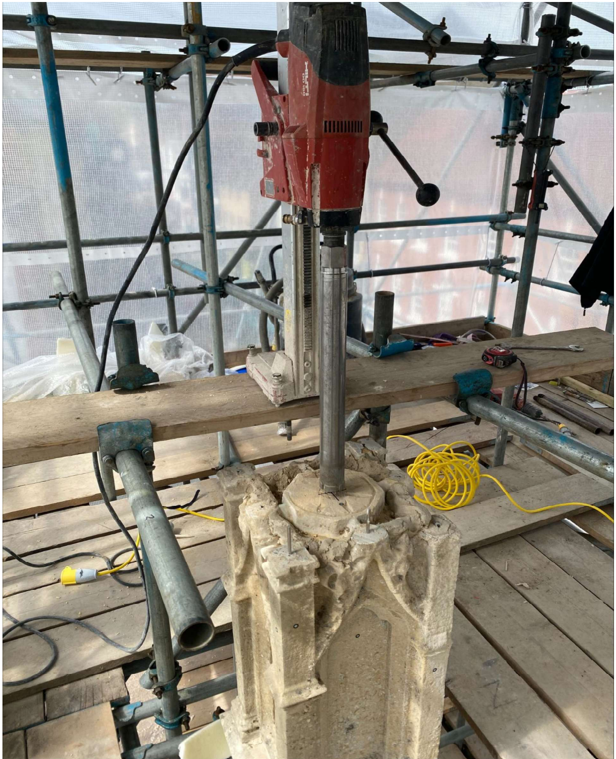
Photo showing core drilling rig to enable precise and careful removal of the ferrous fixings
